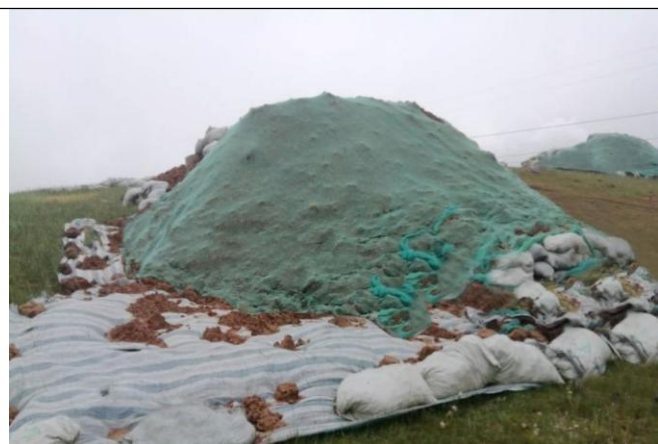
临时铺垫、苫盖、拦挡
